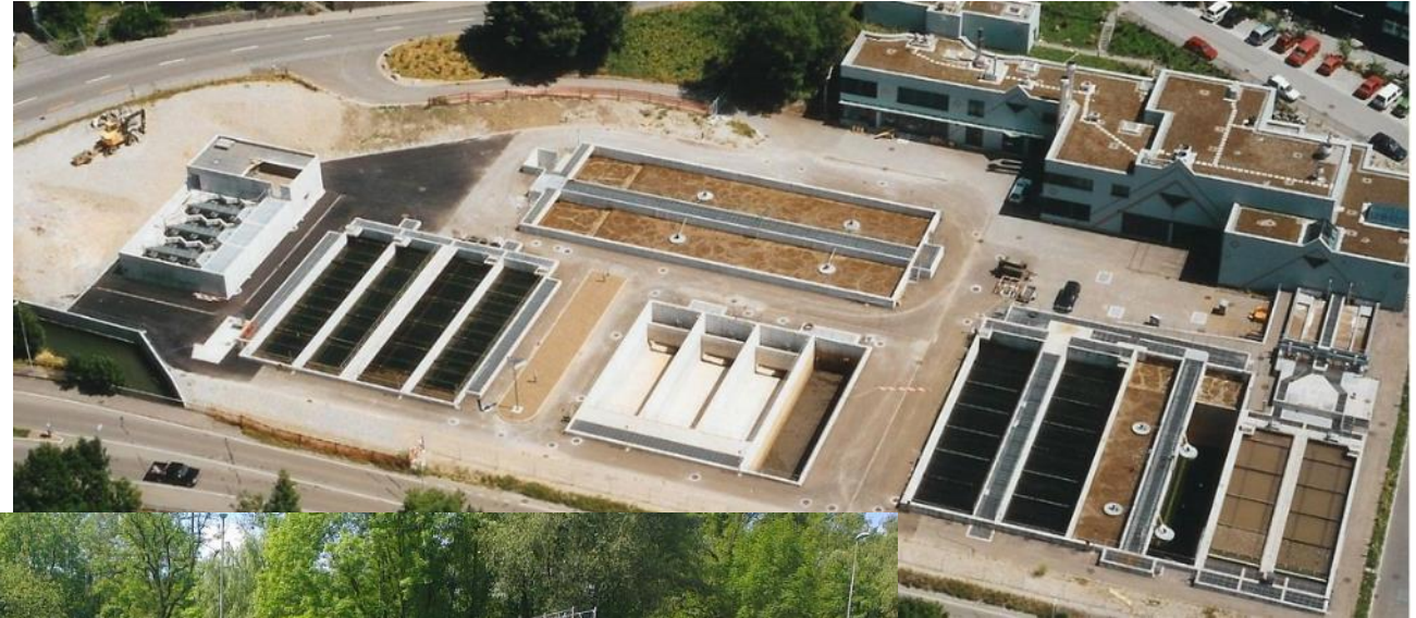
WWTP Flos in Wetzikon
